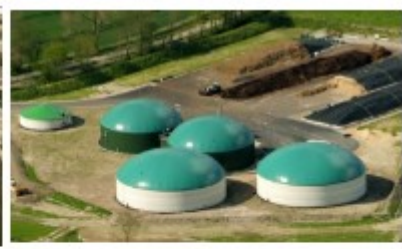
Biogas and AD
